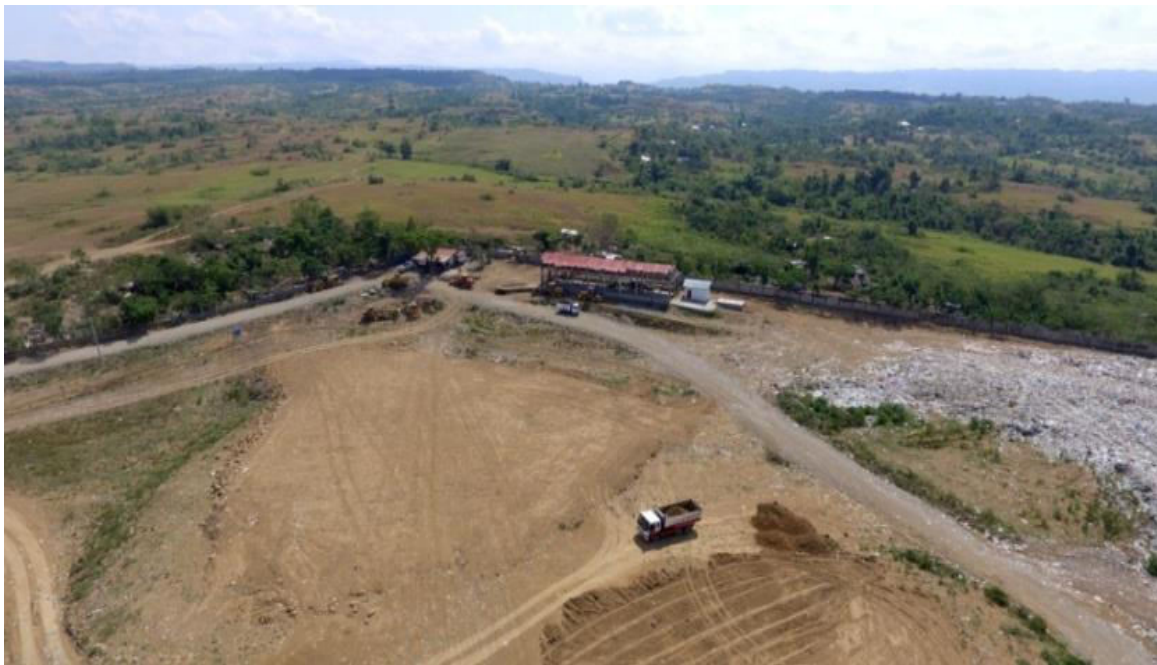
Disposal facility situated at barangay Carig Norte, Tuguegarao city
