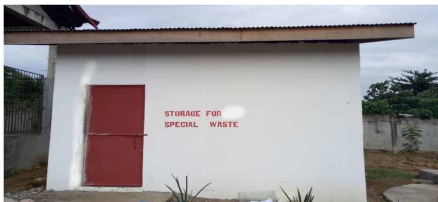
Figure 11. Structure for the Storage of Assorted Special Waste
