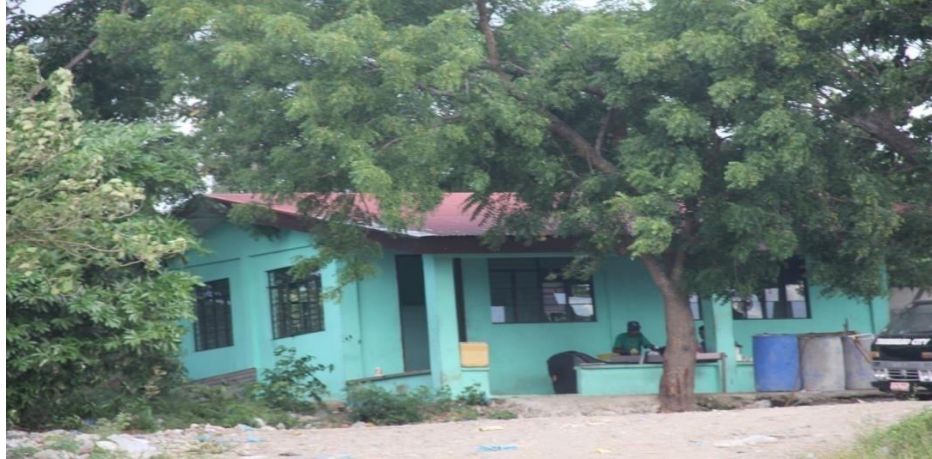
Established administrative building at the Sanitary Landfill
